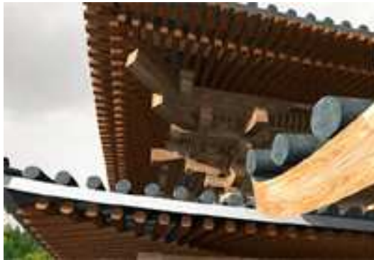
Color schematic of BYODO-IN temple's interconnecting EAVES, BRACKETED COLUMN, and PURLINS which supported the large sloping roof.
