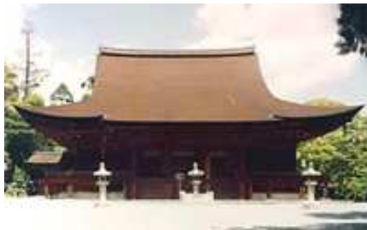
Contoured wooden planks of MIIDERA temple, projecting the flow of a smooth circular arc onto its eaves.
