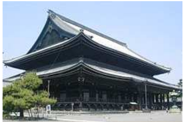
Massive double-level eaves of the HIGASHI HONGANJI temple, constructed on a raised rectangular base in Kyoto, Japan. It was built in 1602 when a schism broke out with its sister temple, the NISHI HONGANJI.
